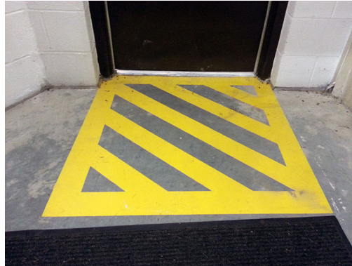
Painted Exit Marking
